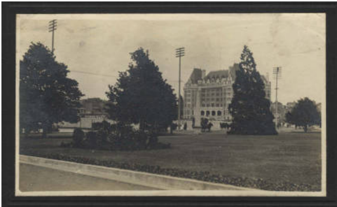
Empress Hotel before 1910 addition, University of Victoria Archives, Frank and Cecilia Sylvester family fonds, AR 281, 1908.
